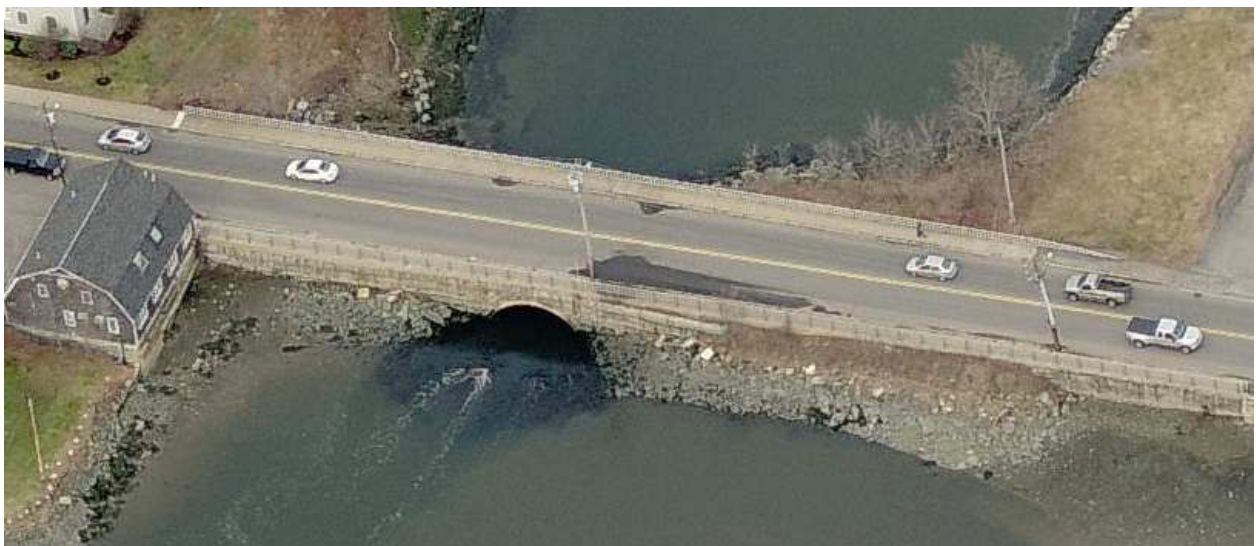
PHOTO 5 Culvert looking north, flood tide, date unknown, courtesy Bing Maps
