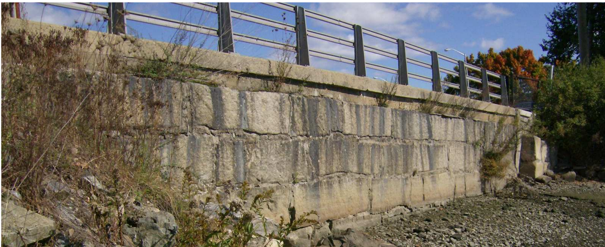
PHOTO 2 Southeastern section of wall looking northeast. Taken 10-14-09 by D. Mellor
